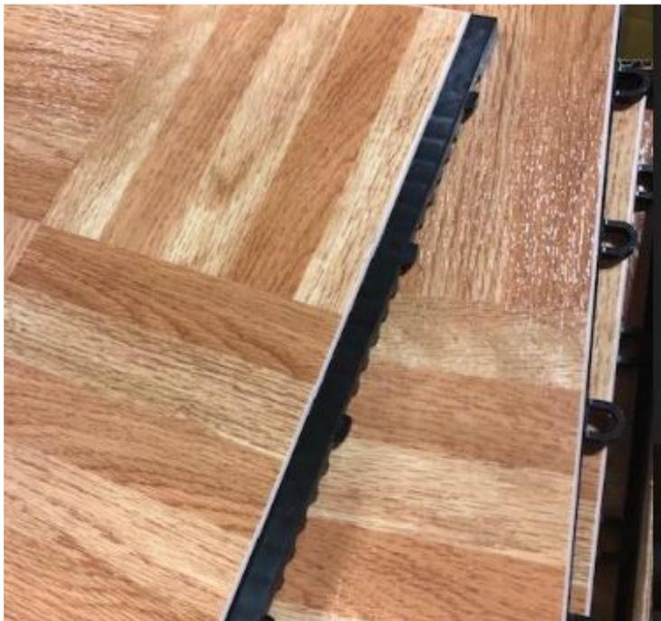
A pressure-sensitive adhesive attaches the wood-look top layer to the plastic base of the tile. If the tiles get hot, the pressure-sensitive adhesive can heat up and loosen, and the top layer can shift when you walk or dance over it.
